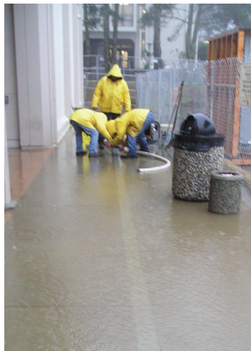
Engineers at Skyline attempt to unclog a flooded drain.
