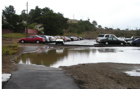
Skyline Parking Lot M flooding.
