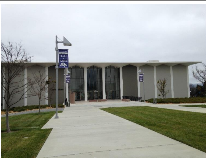
Photograph 11. Gymnasium. View east looking at main elevation and entrance.
