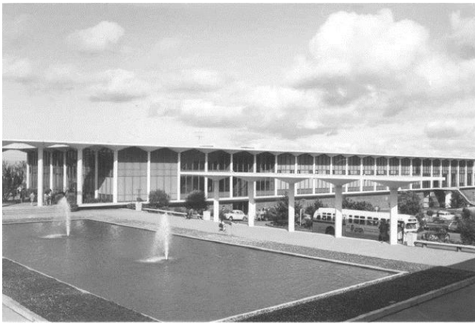
Photograph 19. Art Building and original pool, circa 1964.
