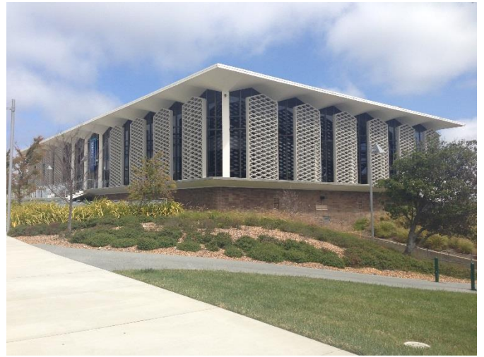
Photograph 5. Library building. View north.
