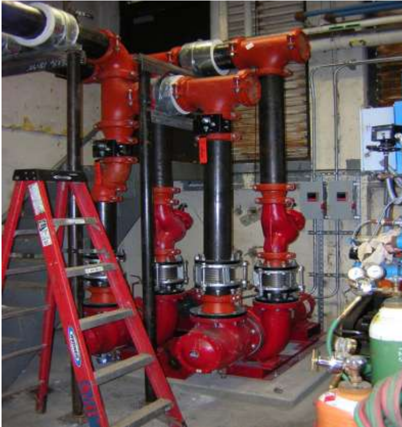
HHW System Conversion (Pumps) at Skyline College
