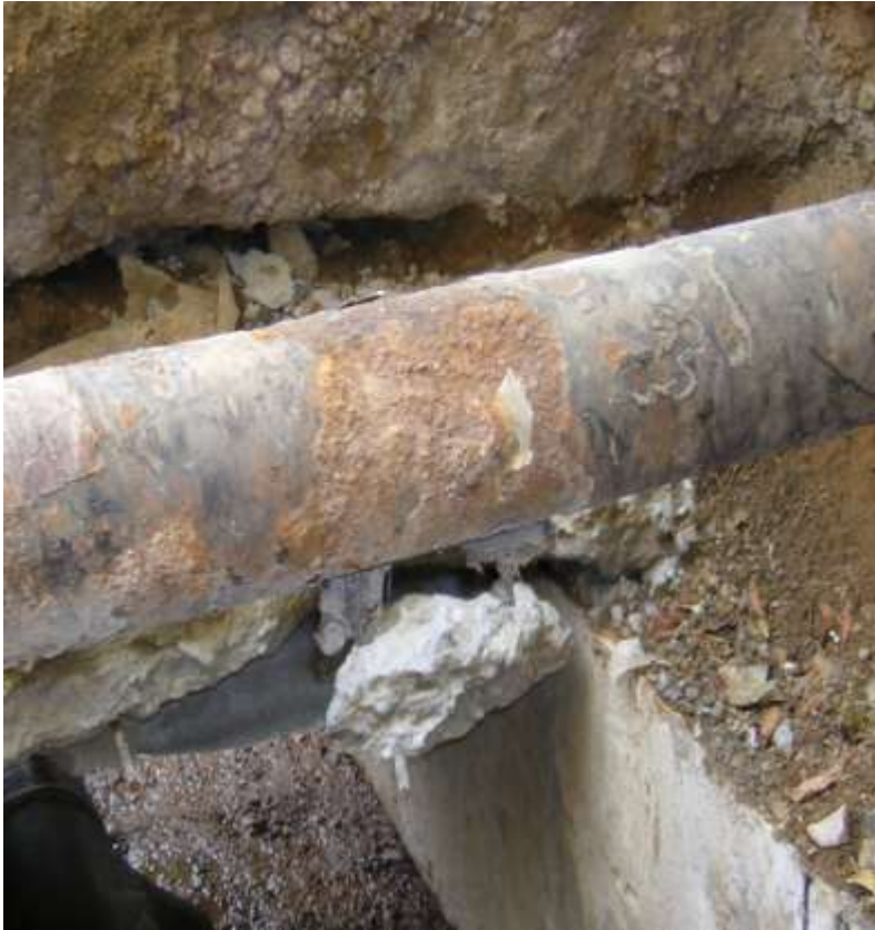
Damaged Piping at CSM & Skyline College
