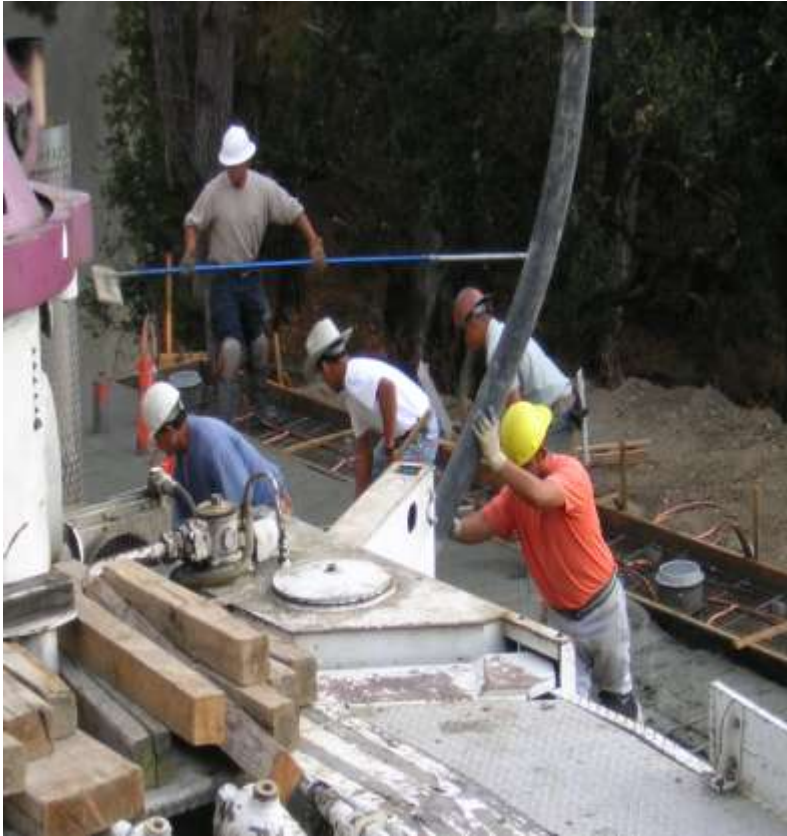
Concrete Pumping & Finished Concrete Pad - CSM
