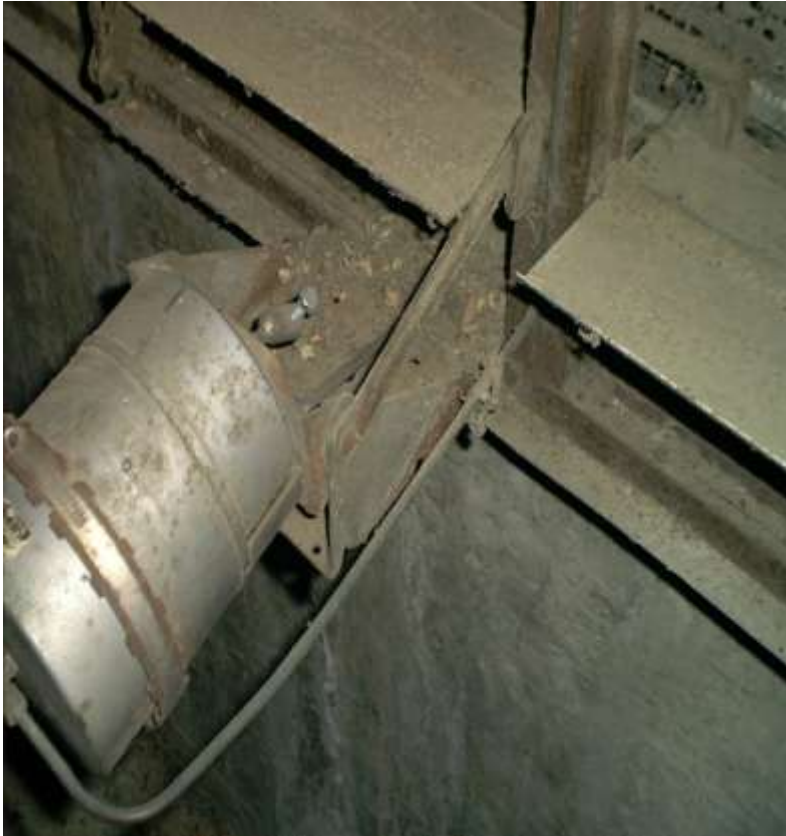
Pre & Post-Retrofit Damper Actuators
