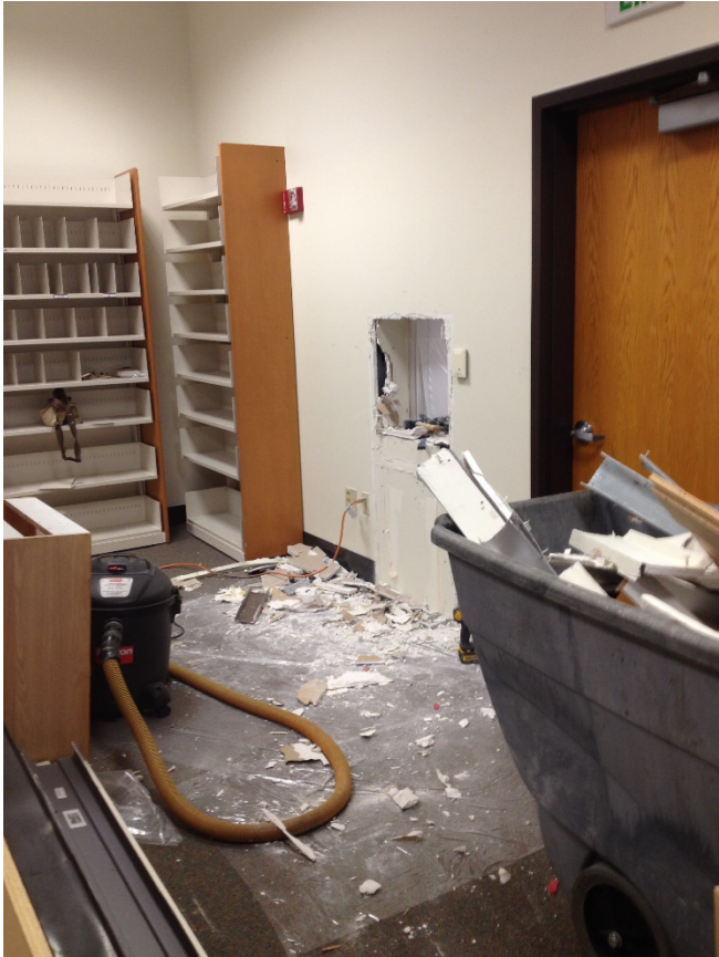
Demolition of unused bookdrop
