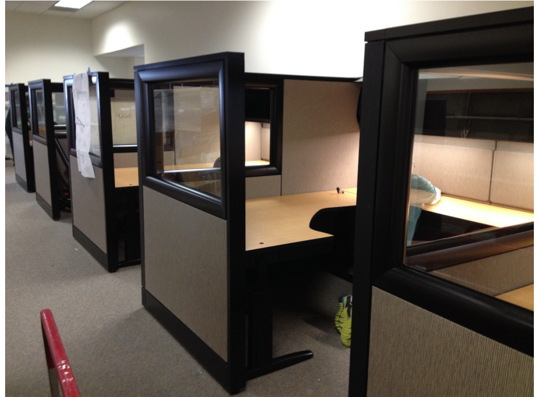
Installation of new cubicles
