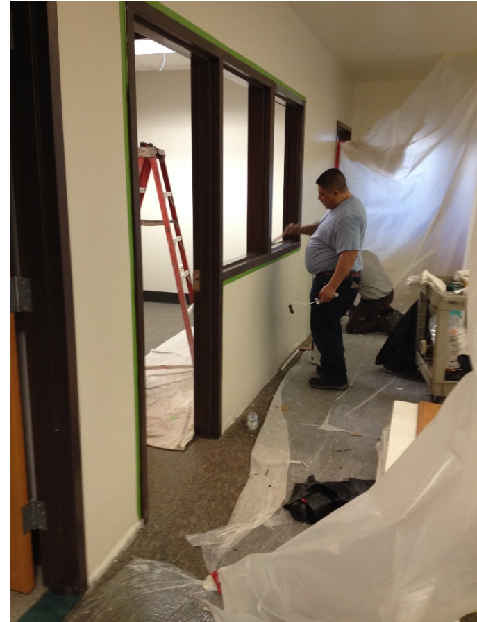
Painting during construction
