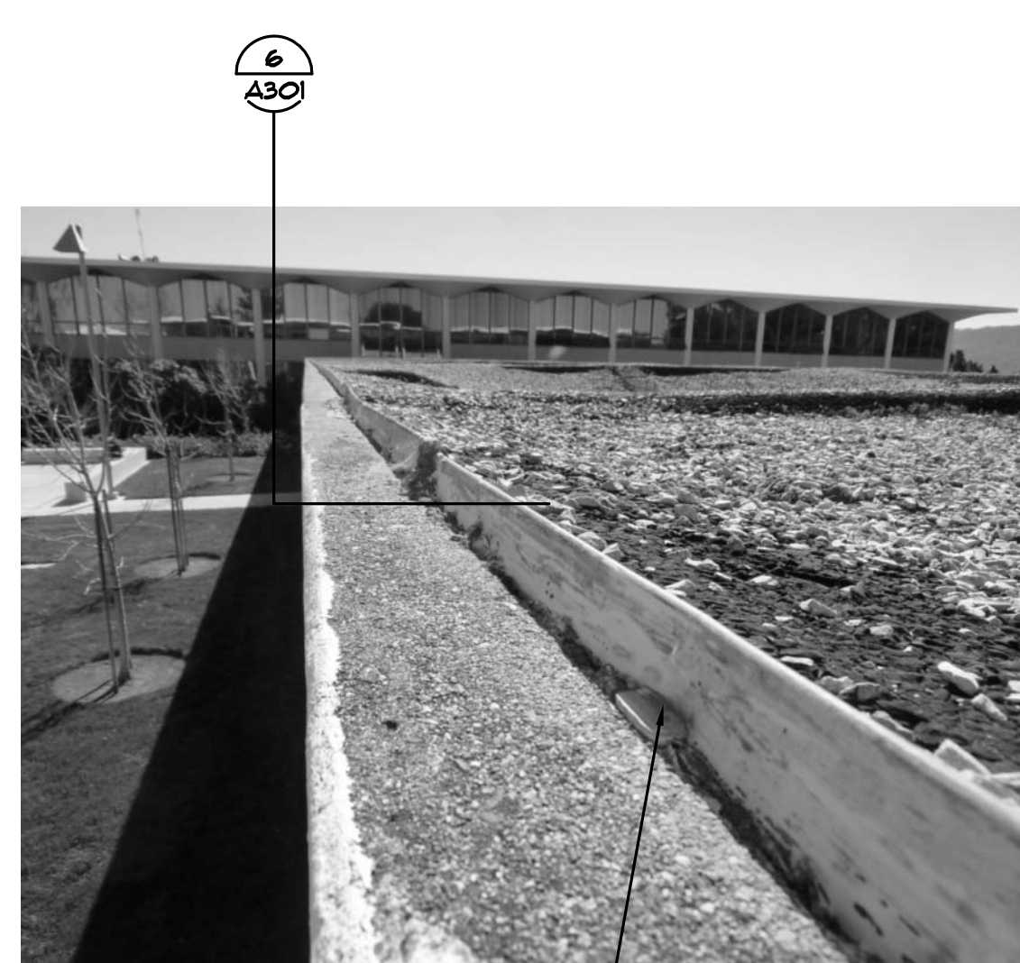
(E) SEALANT AT OUTSIDE EDGE OF METAL FLASHING CONTAINS ASBESTOS. ABATEMENT REQUIRED, FOLLOW ABATEMENT PROTOCOL
