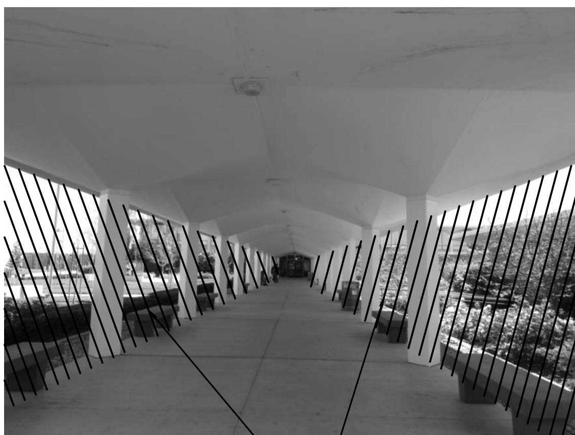
BARRIER FENCING WITH MESH FABRIC AND LOCKS, WHERE POSSIBLE WHILE MAINTAINING ADA ACCESS
