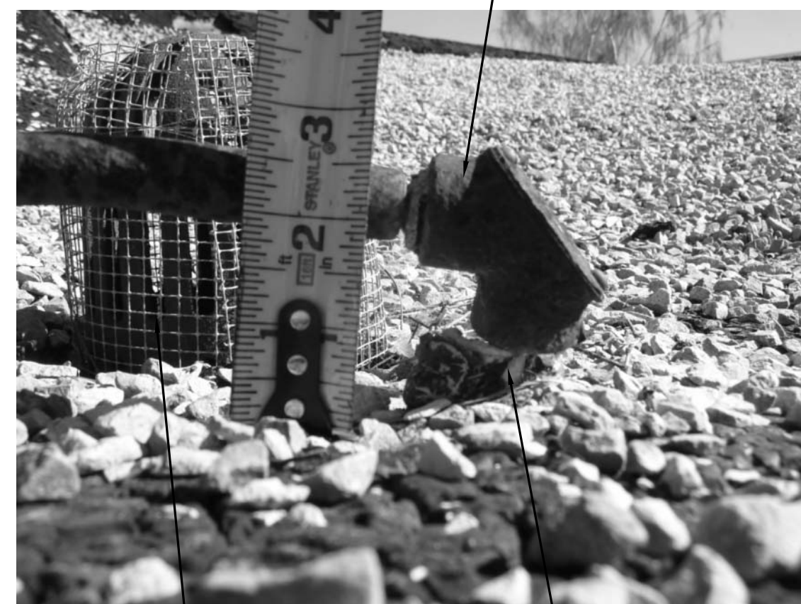
DEMOLISH (E) STRAINER DOME, CLAMPING RING AND BOLTS. SALVAGE COMPLETE ASSEMBLIES AND DELIVER TO OWNER
