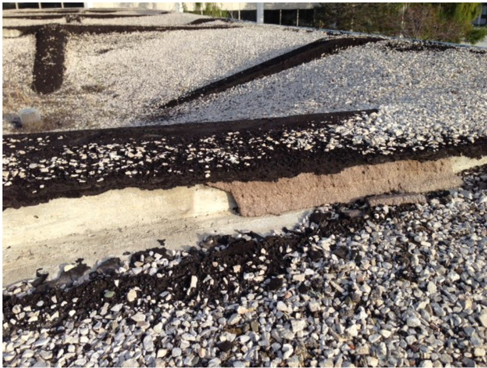
Photo of B14-16 Colonnade Roof Surface
