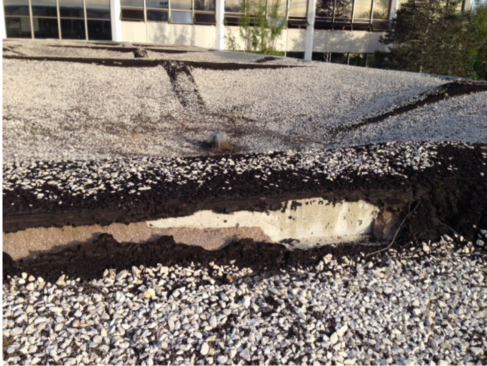
Photo of B14-16 Colonnade Roof Surface
