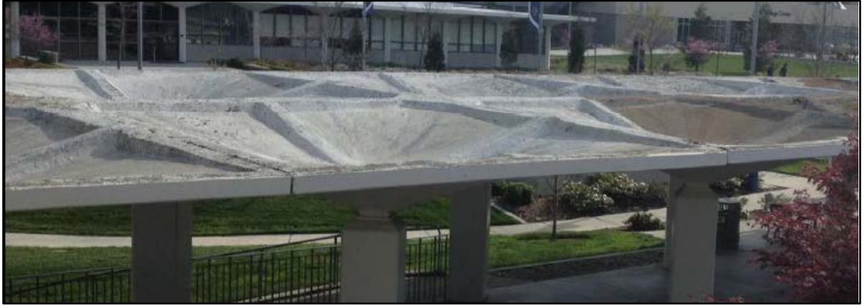
Photograph of B16-18 Colonnades Roof Surface
