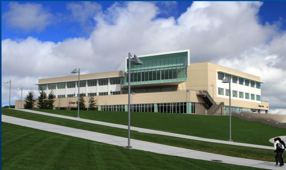
College of San Mateo Building 10 College Center (21.5%)
