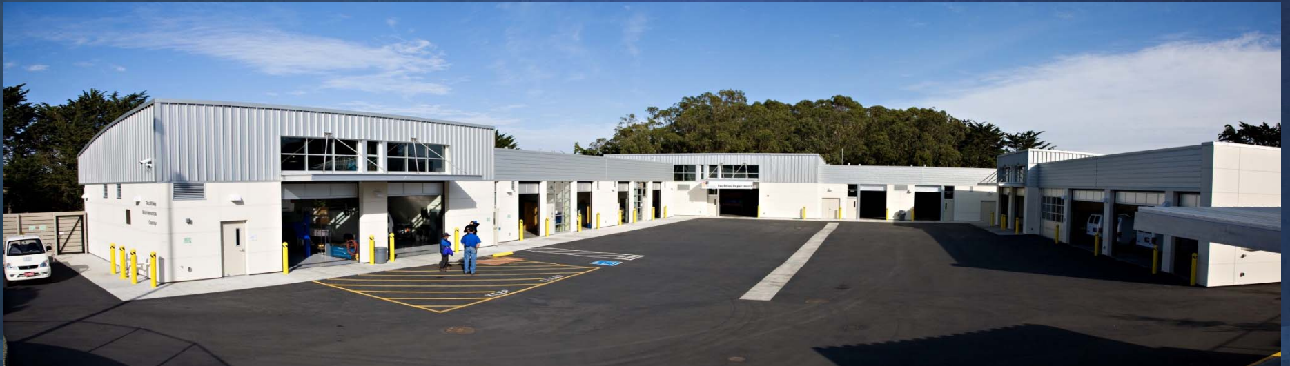
Skyline College Facilities Maintenance Center (FMC) (18.2%) LEED Gold
