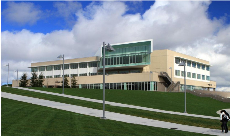
College of San Mateo Building 10 College Center (21.5%)
