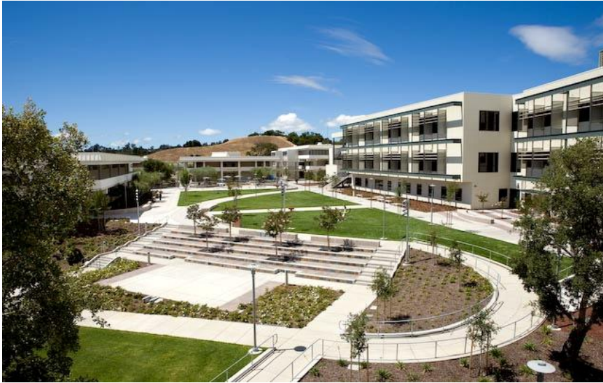
Cañada College Building 9 Library/Learning Resource Center (30%)
