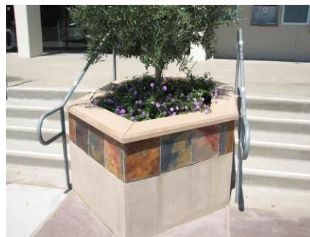
Ambrose stucco sack/patch on formerly aggregate planter
