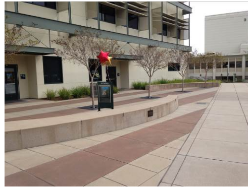
Davis Kahlua concrete bands in natural concrete flatwork at Building 9
