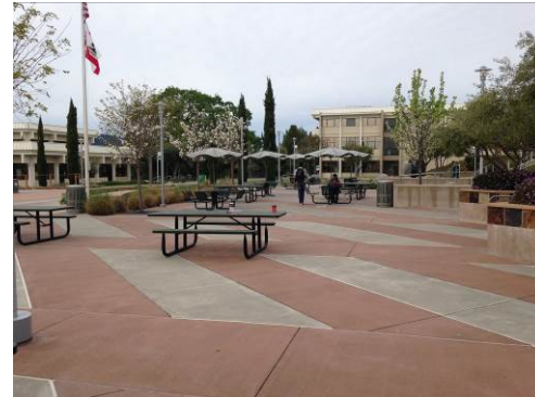
Davis Kahlua concrete bands in natural gray concrete flatwork at Building 2
