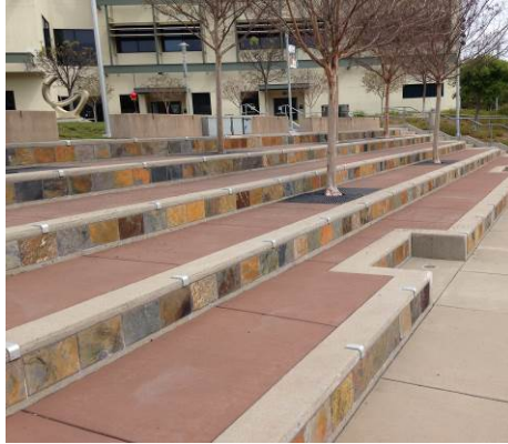
Davis Kahlua concrete at Amphitheater (with African multicolor slate)
