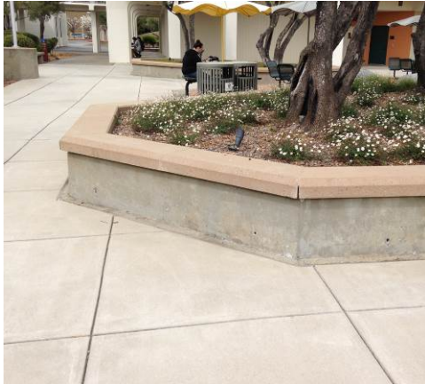
Pre-cast Davis Sandston sandstone cap on retrofitted planter by Building 17
