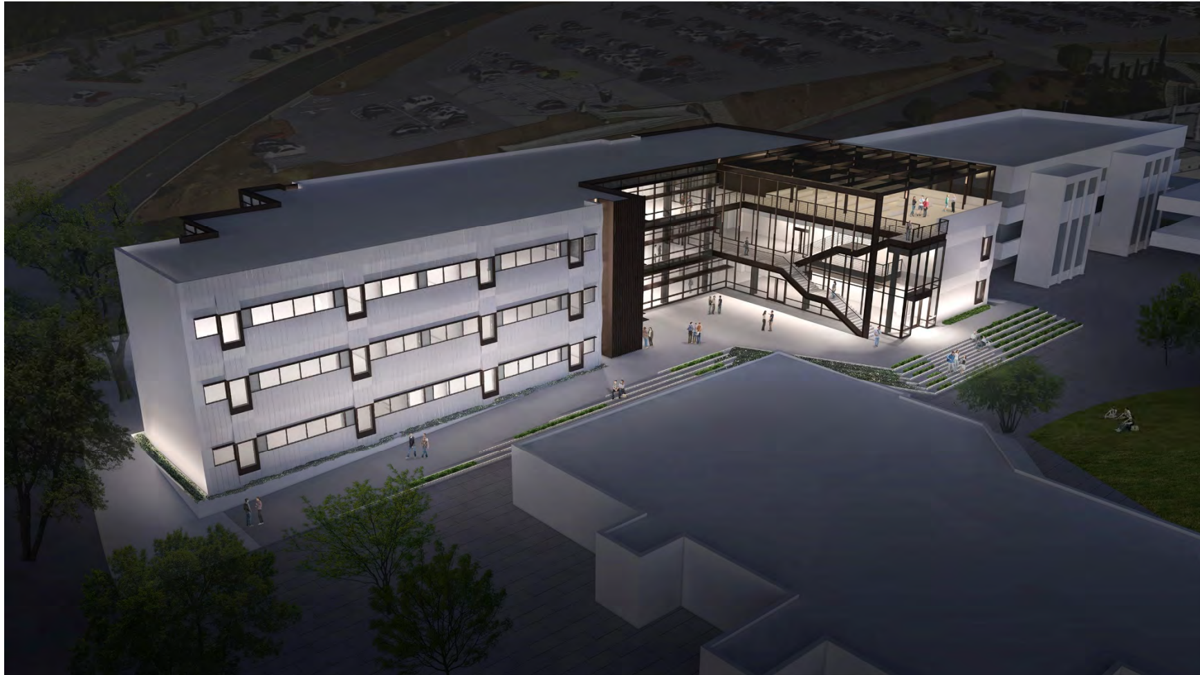
Cañada College Math and Science Building (B23N) [McCarthy/HGA]
