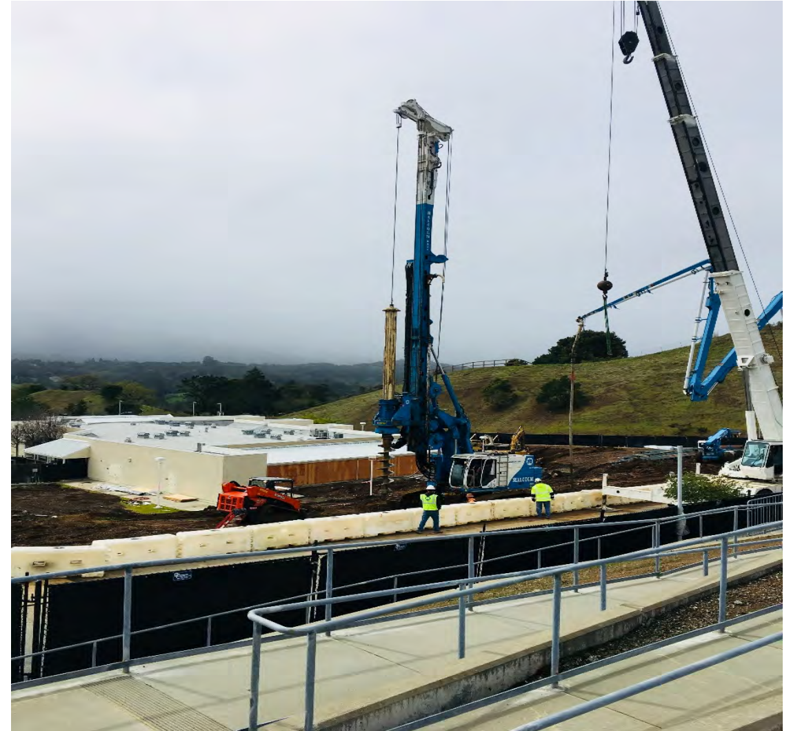
Soldier piles being driven in preparation for retaining wall
