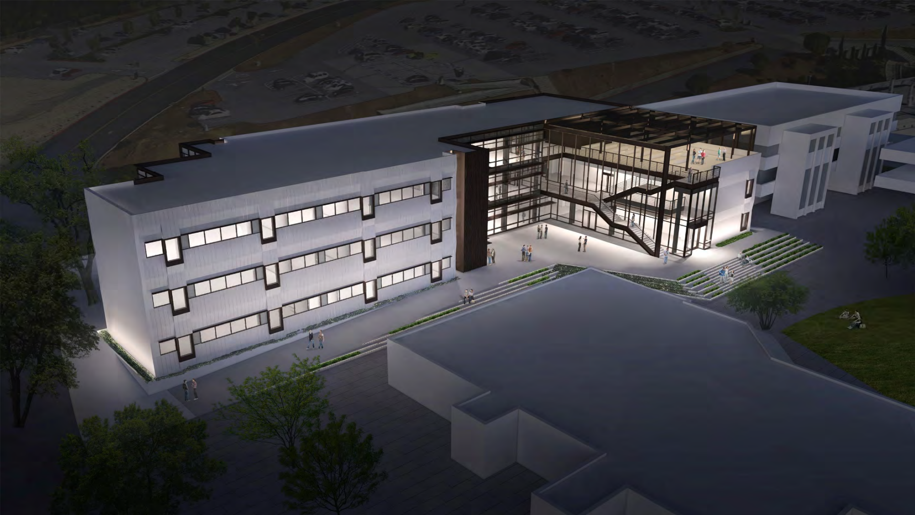
Cañada College Math and Science Building (B23N) [McCarthy/HGA]
