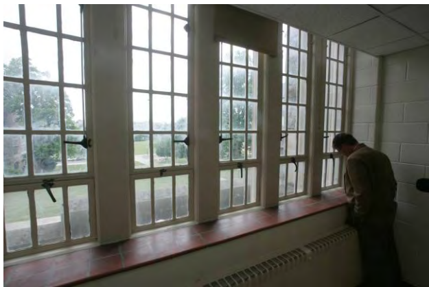
Figure 11. Typical Set of Windows in Norris Hall
