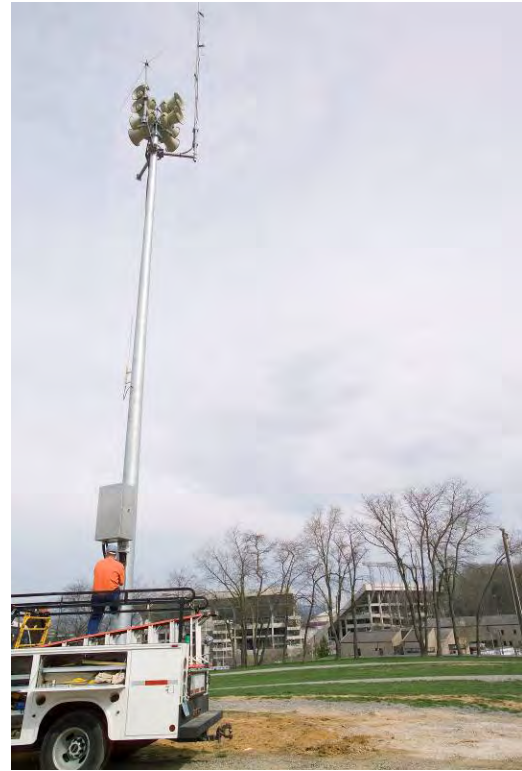
Figure 2. One of the Six Sirens Being Installed on Virginia Tech Campus
