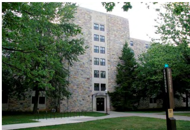
Figure 3. Exterior of West Ambler Johnston
