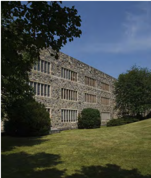
Figure 10. Norris Hall Classroom Windows, Grassy Side
