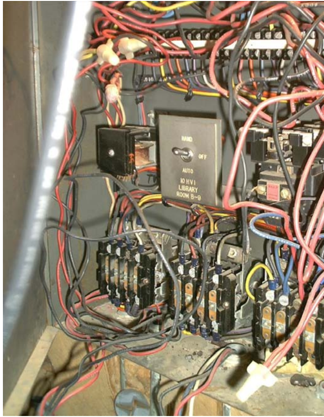
Fig. 1-3: Manual Override on Older EMS Controls
