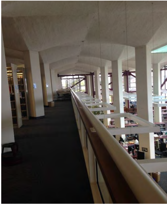
Photograph 9. Library interior. View of two-story colonnades.
