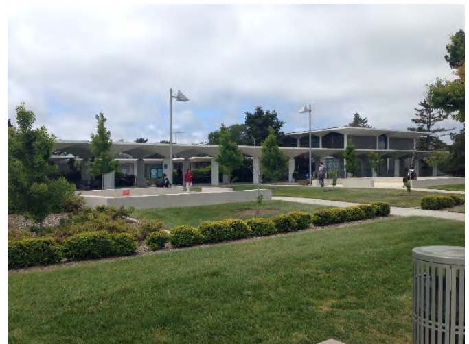
Photograph 16. View northwest at colonnade and building 18. Building 17 is recessed behind the colonnade.
