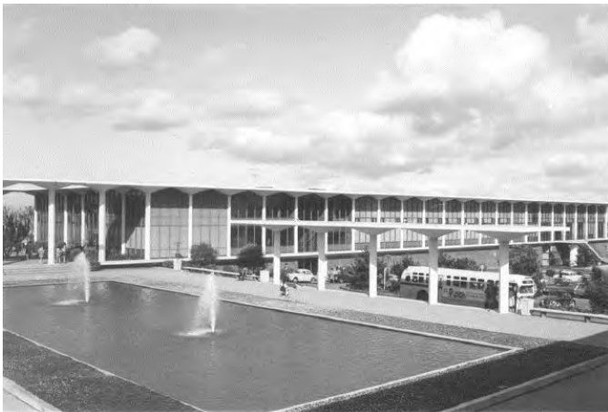
Photograph 19. Art Building and original pool, circa 1964.
