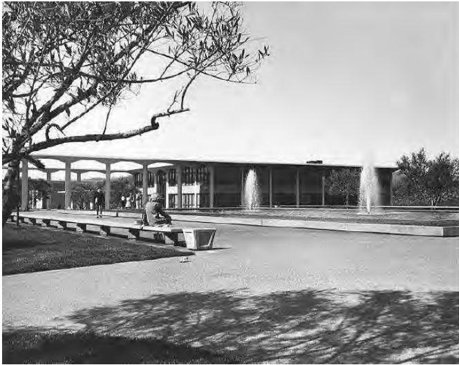
Photograph 25. Admin Building 1, view west, showing original concrete colonnade attached to building 1 and 5. 1965. Circa 1965.
