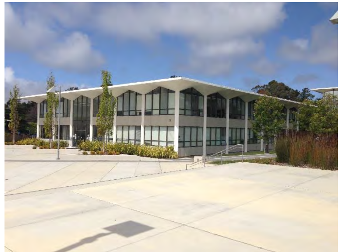
Photograph 10. Building 1. View west looking at main elevation and entrance.
