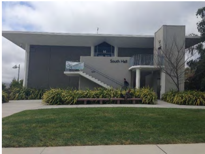
Photograph 15. Building 14, view west showing narrow elevation. Façade similar to building 16 and 18.
