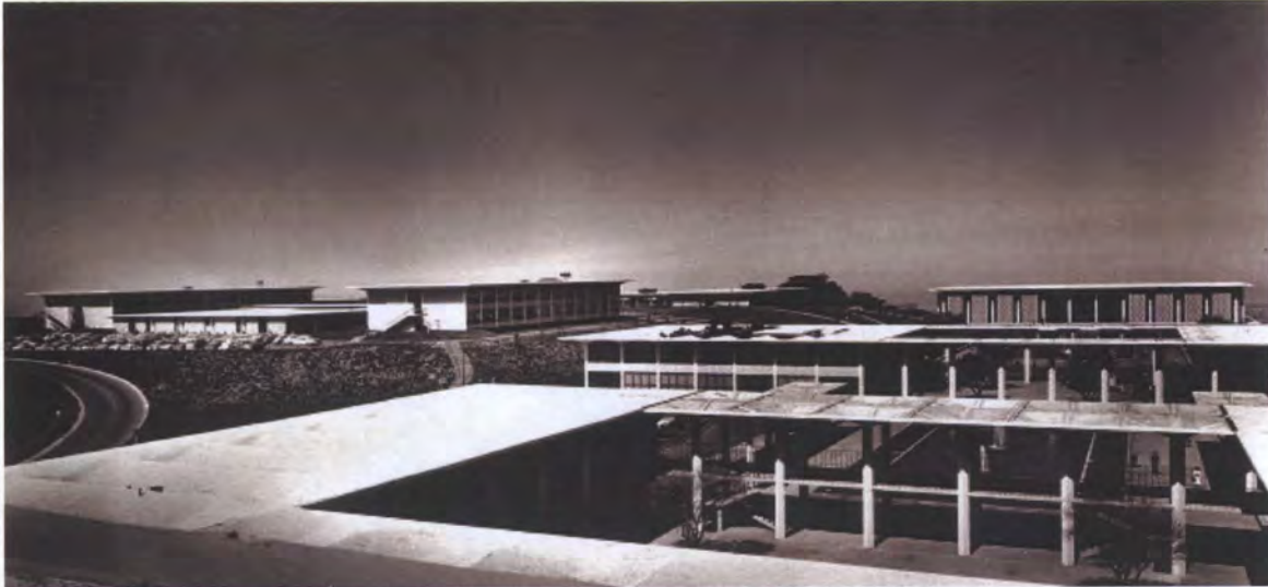
View of the campus, circa 1964, looking at Buildings 14 and 16 on the left and the Library (Building 9) on the right (courtesy College of San Mateo Archives, Historical Photograph Collection)
