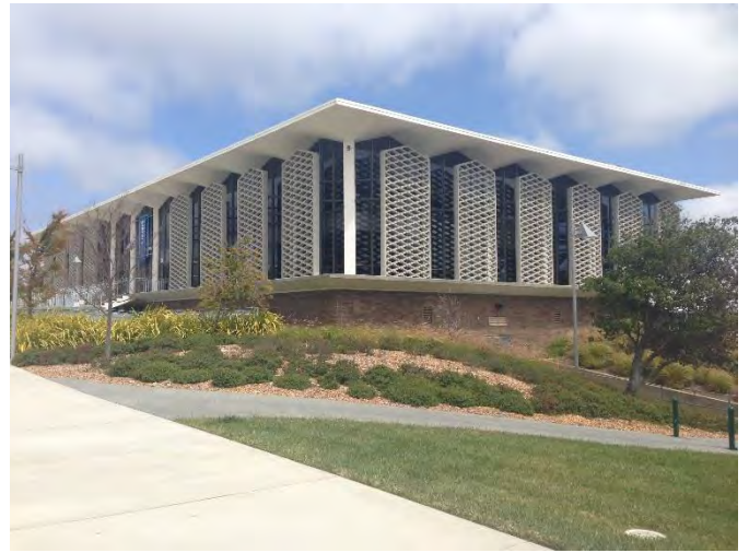
Photograph 5. Library building. View north.
