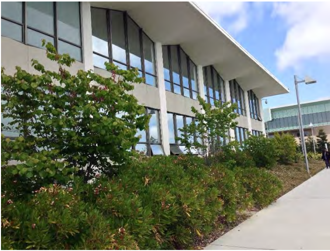
Photograph 17. Building 14 view north. Example glass curtain wall facade.
