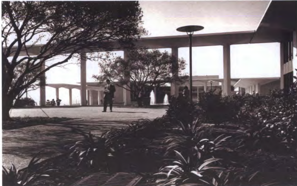
Fine and Performing Arts Center Building, 1970 (courtesy College of San Mateo Archives, Historical Photograph Collection, Photograph #000497).
