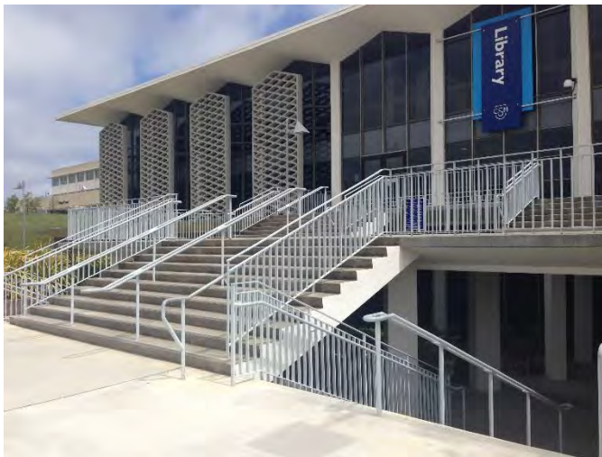
Photograph 7. Library building. View north at main entrance and below grade level.
