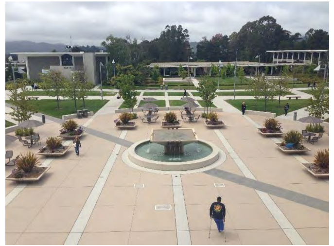
Photograph 18. View looking west from building 10 showing buildings 14-16 and the newly redesigned courtyard.
