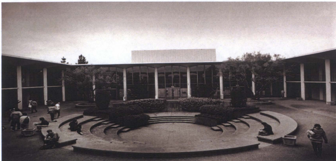
Fine and Performing Arts Center view through the plaza early 1960s (courtesy College of San Mateo Archives, Historical Photograph Collection, Photograph #000497).
