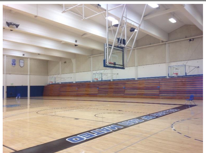
Photograph 12. Gym interior showing roof beams and folded plate design.
