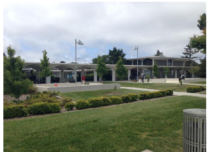
Photograph 16. View northwest at colonnade and building 18. Building 17 is recessed behind the colonnade.
