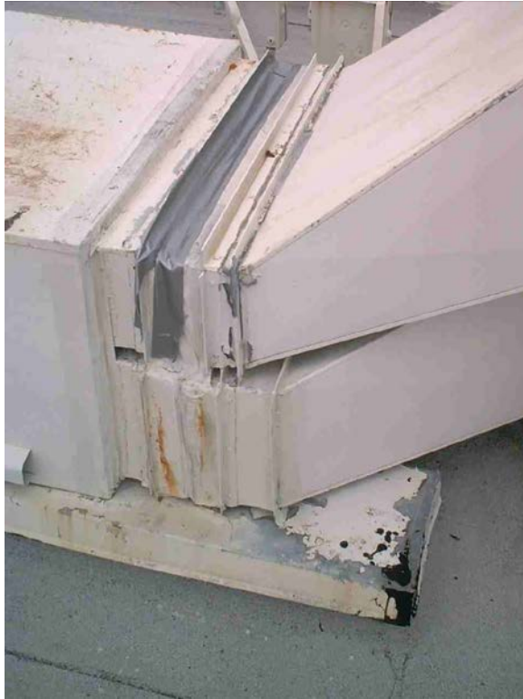
Typical Temporary Duct Repairs
