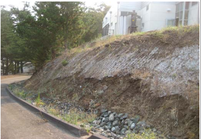
6- Roof drain box - North Slope
