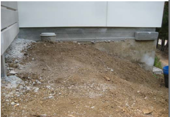
12- Roof drain box - North Slope
