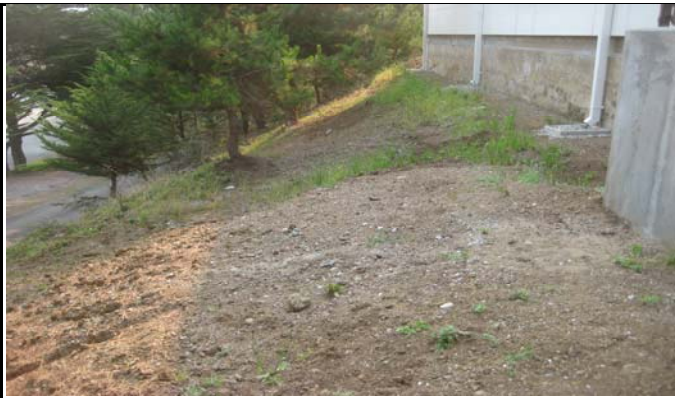
7- Slope to the north
