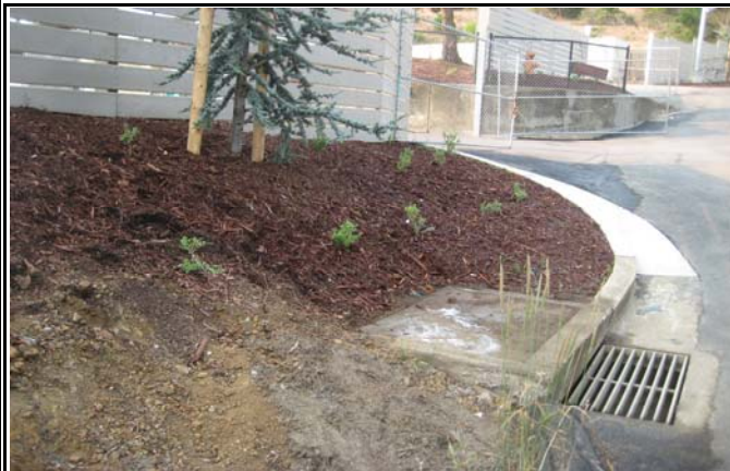
13- Catch Basin On The North Side
