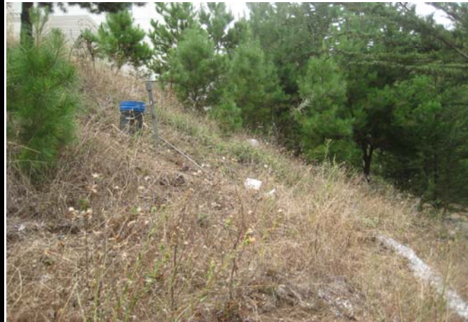
23- Slope erosion on the east
