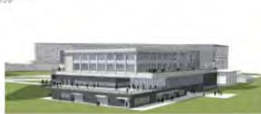
07 South and East Elevations
