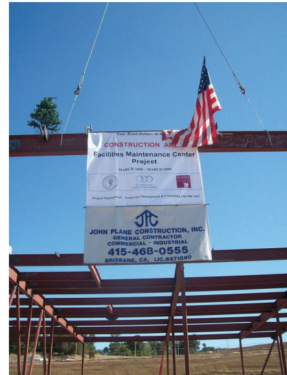
Cañada FMC "Topping Off" Ceremony
