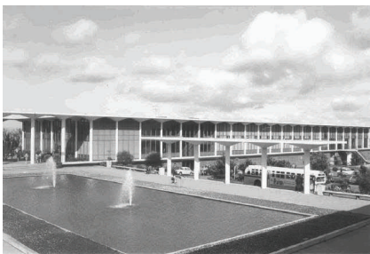
CSM Bldg. 5/6 in the 1960s
