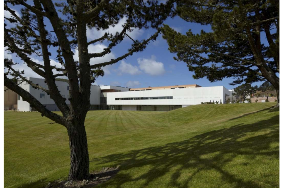
Campus Administration, Cosmetology, & General Classroom Building
