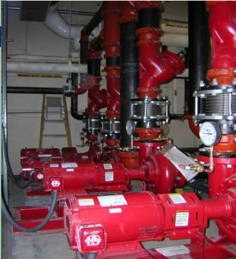
Heating Hot Water Pumping Systems + VFDs
