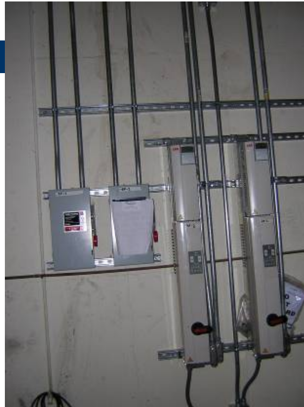
Heating Hot Water Pumping Systems + VFDs
