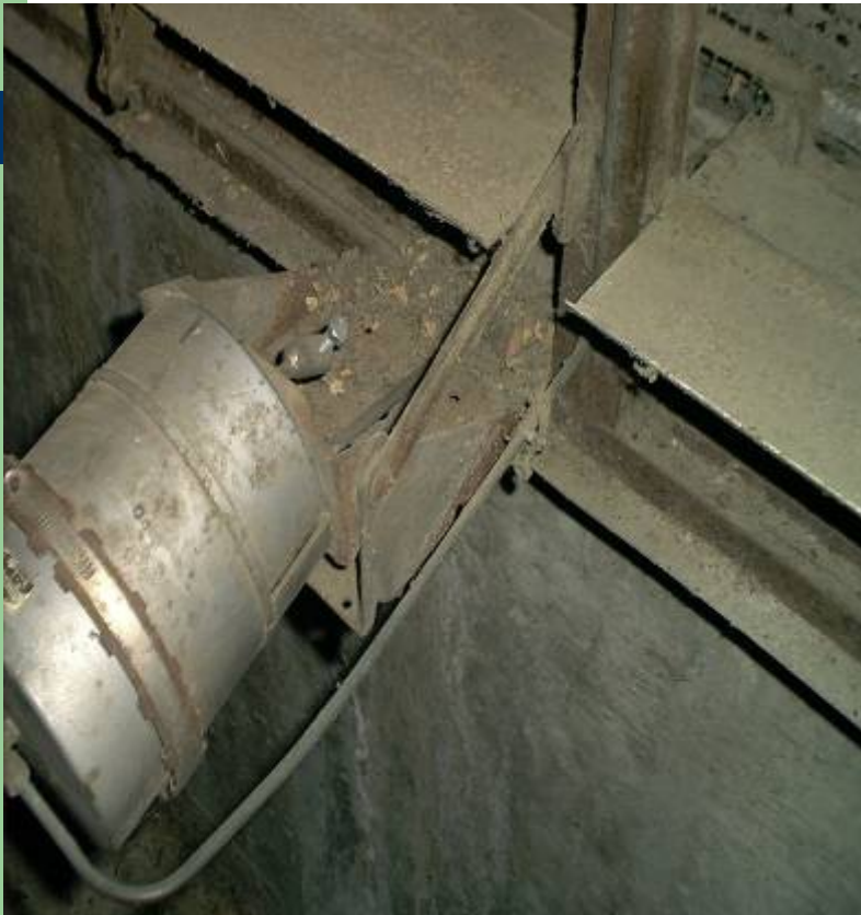
Pre & Post-Retrofit Damper Actuators
