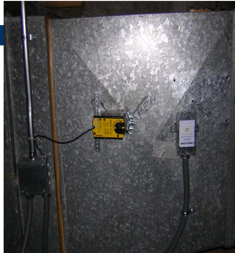
Pre & Post-Retrofit Damper Actuators
