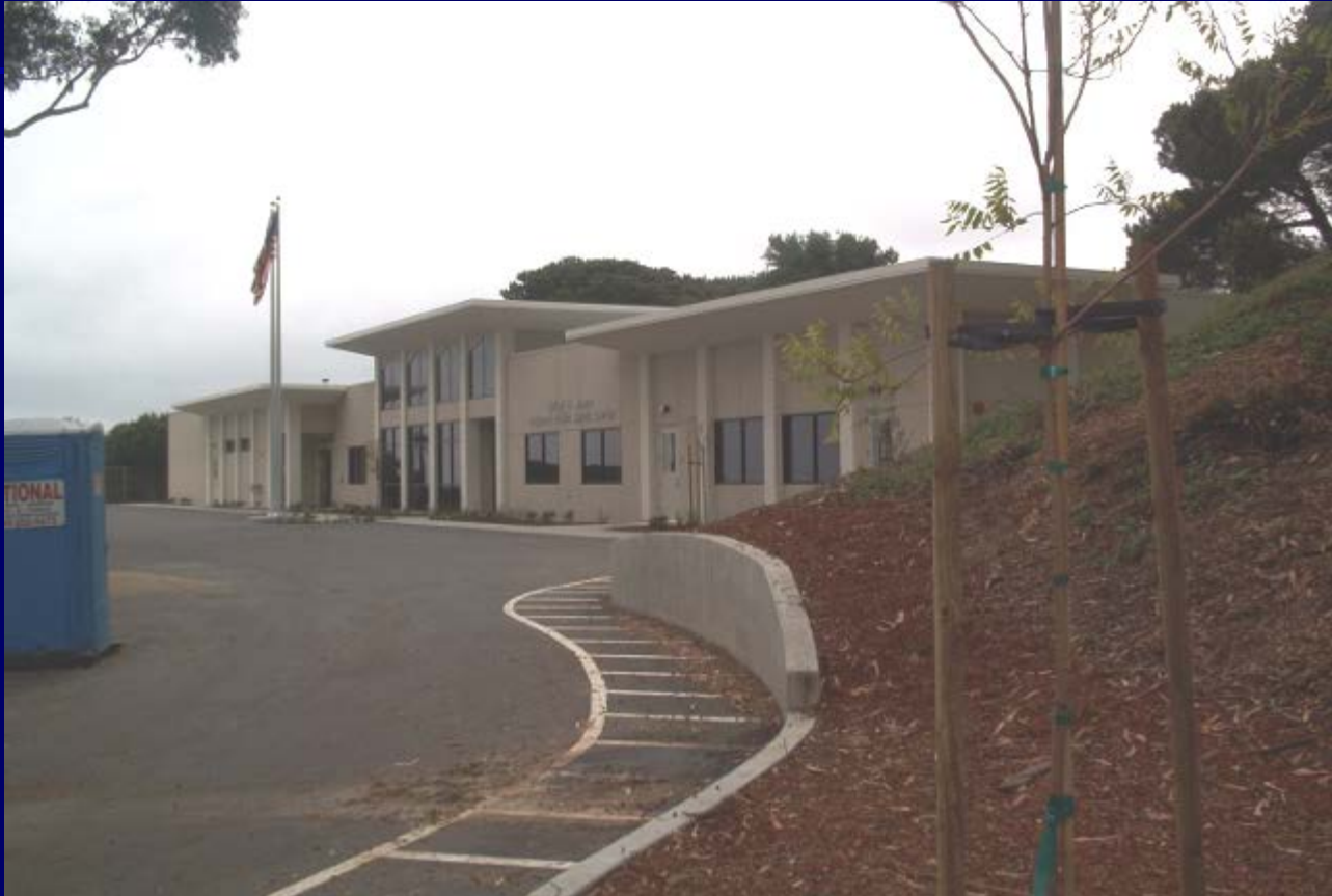
Building 35 – Gordon H. Moore Regional Public Safety Center
