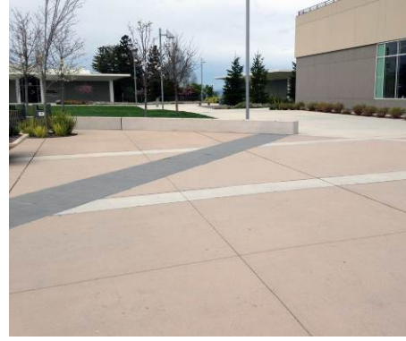
Gibraltar Paver (gray) running through a field of Solomon Canvas concrete with narrow natural gray concrete bands at Building 10
