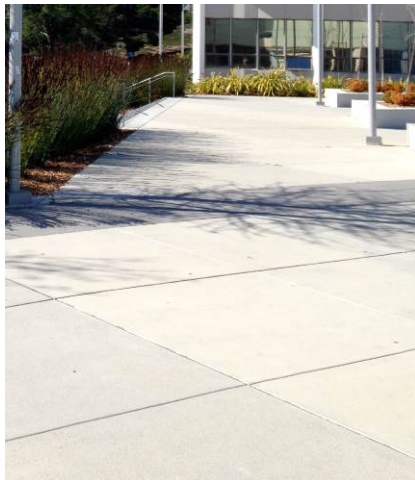
Natural gray concrete with bands of medium broom finish (light) and medium sandblast finish (darker)
