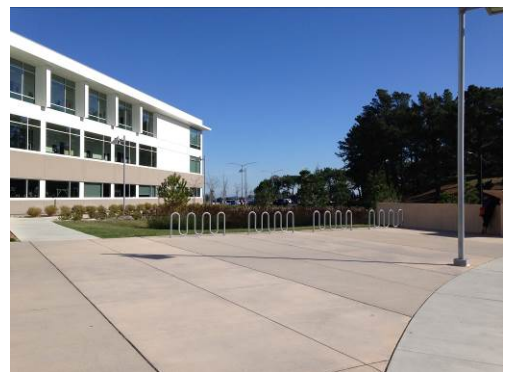
Solomon Canvas concrete with bands of medium broom finish (light) and medium sandblast finish (darker) at Ceremonial Circle/Building 5
