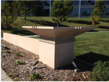
Site wall with Pilaster by Building 5
