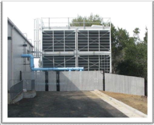
CSM Chiller Plant
