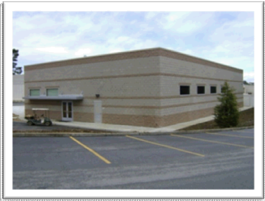
Skyline College Building 11, Automotive Transmission
