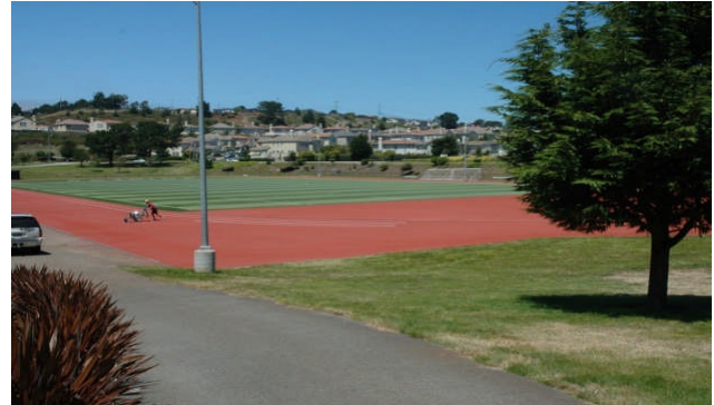
Skyline College Track Resurfacing
