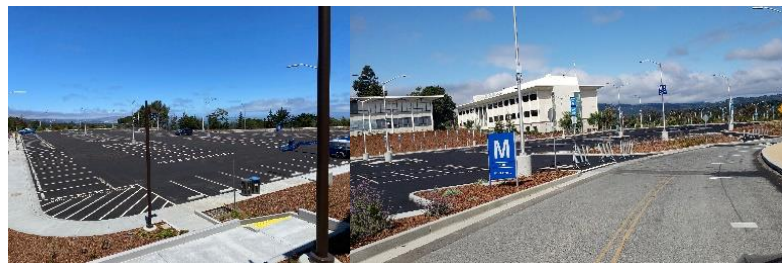
Building 20 Demolition / Edison Lot 7 Expansion
