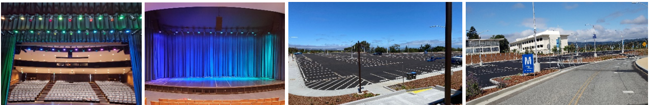
Building 3 Theatre Modernization
