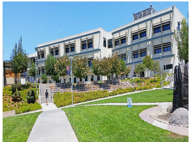
Canada Building 9 Library, Learning Center
