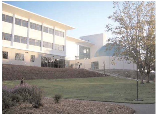
CSM Science Building - Bldg. 36 (South view)
