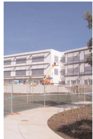
Cañada Building 9 Under Construction
