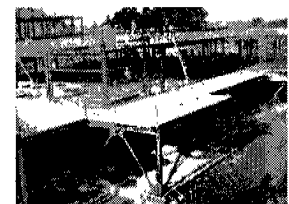
Skyline Building 6 & 7 Under Construction
