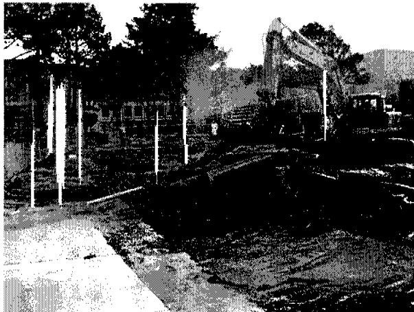
Demolition Work for New Skyline Student Union Building/Science Wing
